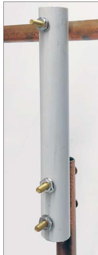
Figure 7 — Mounting brace location.
